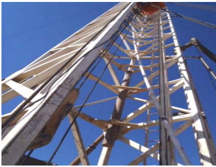
ASPC-Lewis Drill New Water Well #5 Rig Set Up for Drilling
