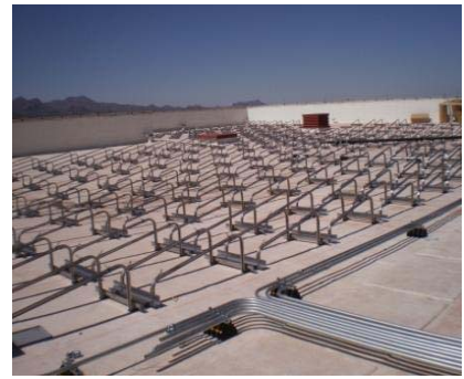
Tucson Office Complex Solar Photovoltaic Install
