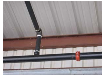
ADOT Mesa Equipment Services Fire Sprinkler & Alarm Install
