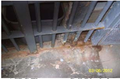
ASPC Florence – Cell Block 2 Structural Repairs
