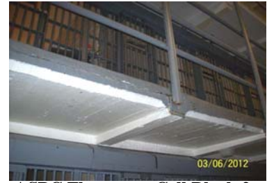
ASPC Florence – Cell Block 2 Structural Repairs
