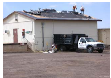
ADOT Show Low Maintenance Yard Roof Replacement
