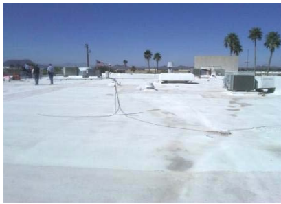
DPS Statewide Roof Replacement Tucson, AZ
