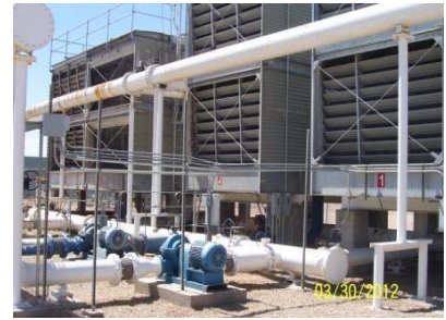
Arizona State Hospital, Phoenix, AZ Cooling Tower Repair & Replacement
